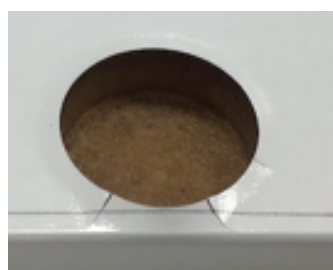
Cracks on top surface only (pass)
