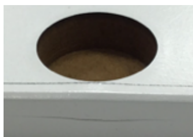
Cracks on edge (fail)
